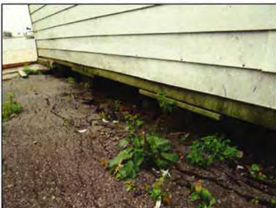
Figure 106: Wood footings beneath the Workshop.
