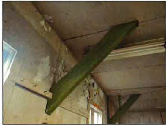
Figure 91: Detail of the bracing in the Workshop.
