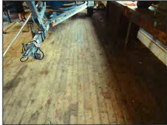
Figure 89: Detail of the wood floor.
