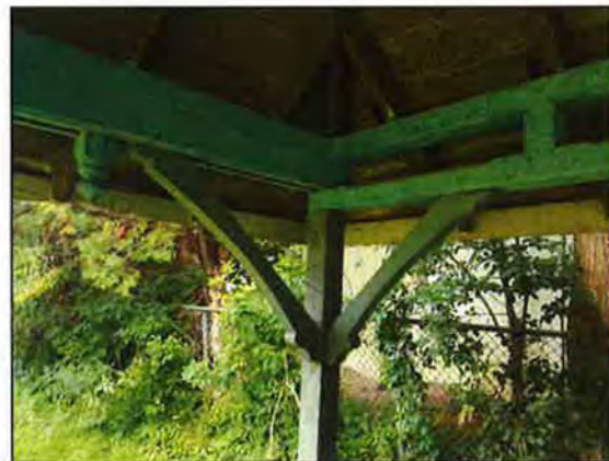
Figure 119: Truss and brace system.
