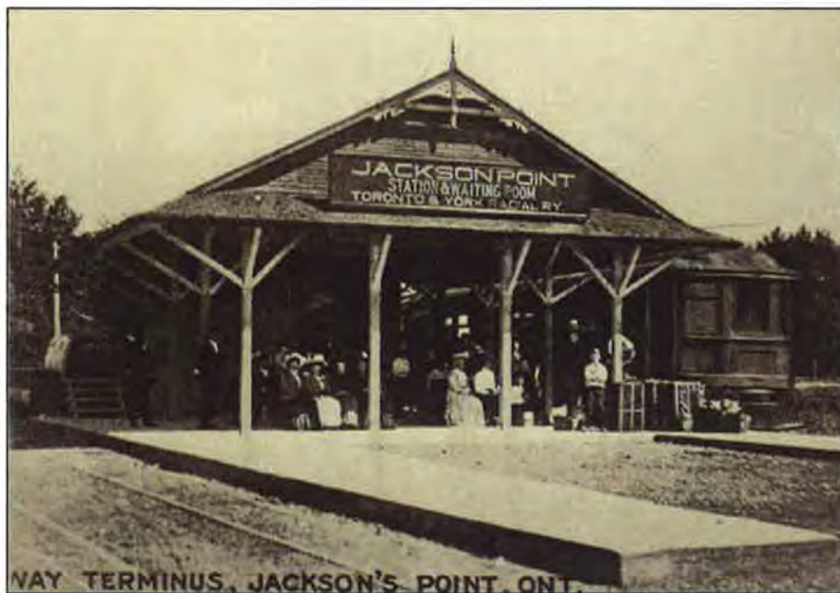
Figure 13: Jackson's Point Radial Railway Station (Toronto Library 976-21-10)
