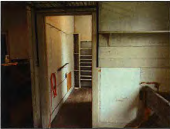
Figure 90: Office space within the Workshop.
