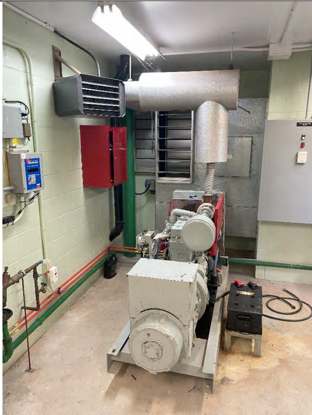
Sewage Pump Station Back-up Generator
