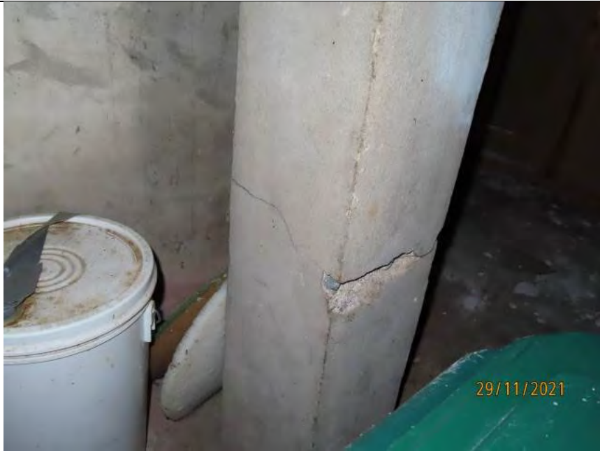
Belhaven Hall damaged column
