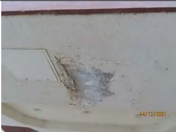
Damaged soffit and flat roofing – Pepperlaw Lions Hall Canopy
